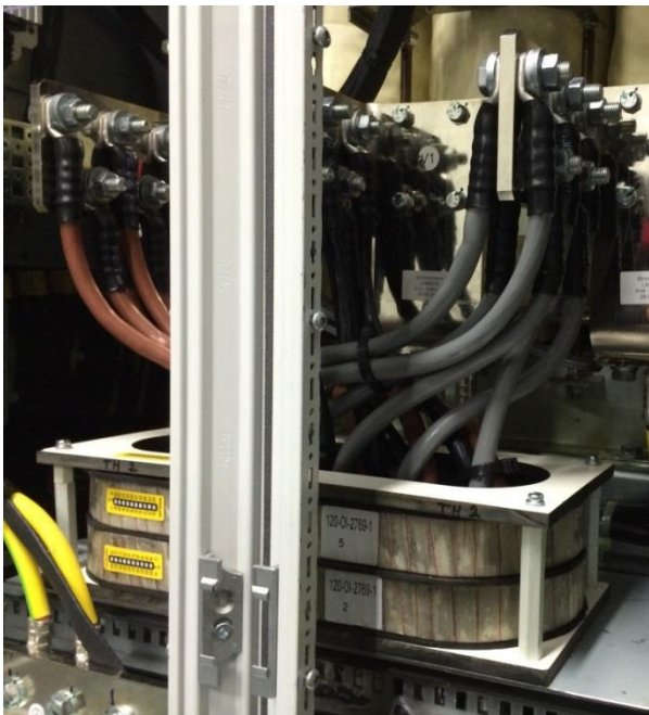
Fig. 5: two assembled cores in the cabinet
